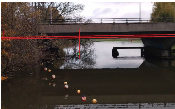
Figure 6. Vertical reference beneath a pipe under a bridge. The feature is below the pipe and bridges the difference from the surface water to the pipe and above the pipe to the bridge surface (in the case the pipe is viewed from the bridge surface).
